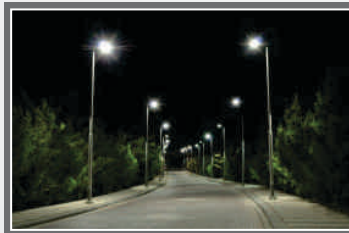
SOLAR STREET LIGHTING
